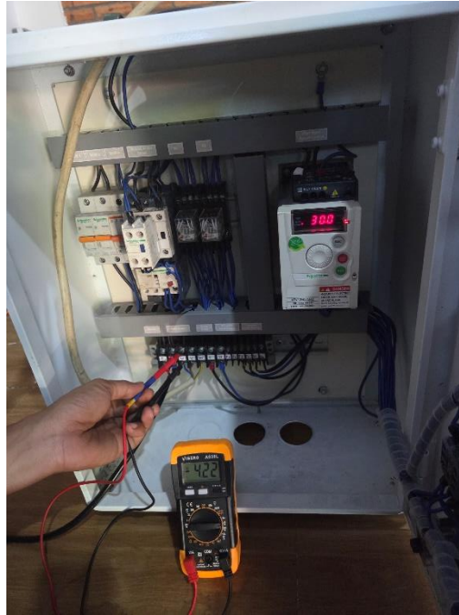
Figure 3. Initial Testing of Forward Rotation Configuration
