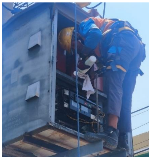
Figure 3. Dust and Rust Cleaning
